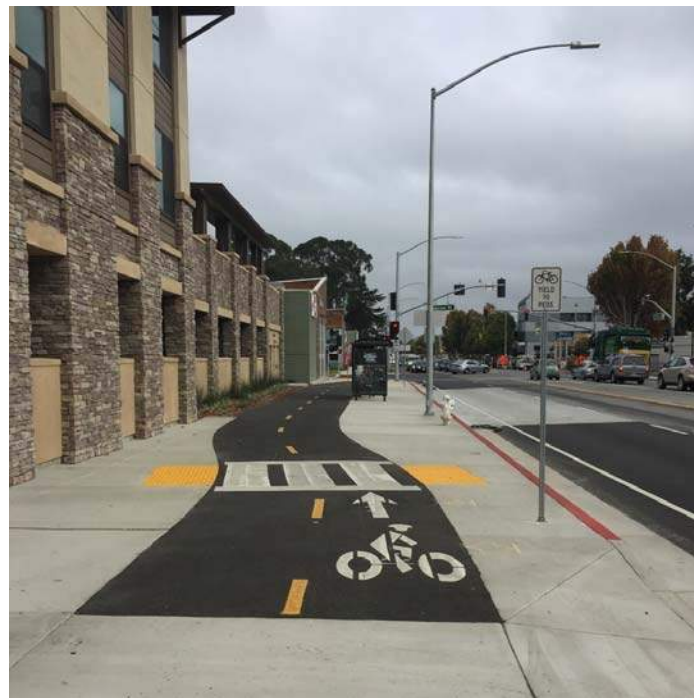
An example of a two-way raised cycle track adjacent to a bus stop and shelter in the City of Albany along San Pablo Avenue.
